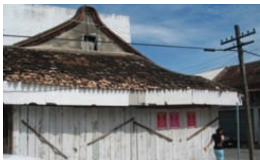
Figure 16 A first unit of nine row houses at Nang-ngam Road.
