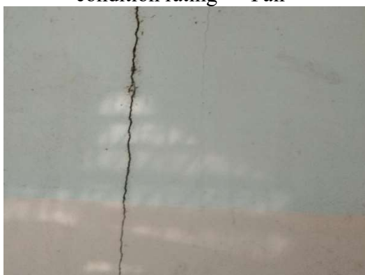
F-03: Vertical crack on wall ( w=0.2 mm), condition rating = “Fair”
