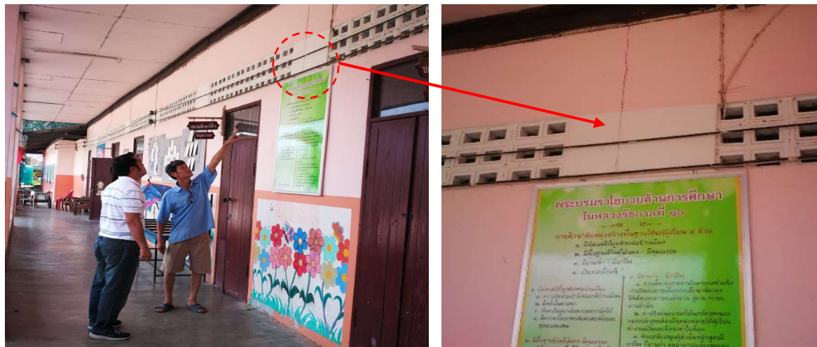
Figure 3 Walk-through preliminary inspection of damaged building (photo no. F-01)
