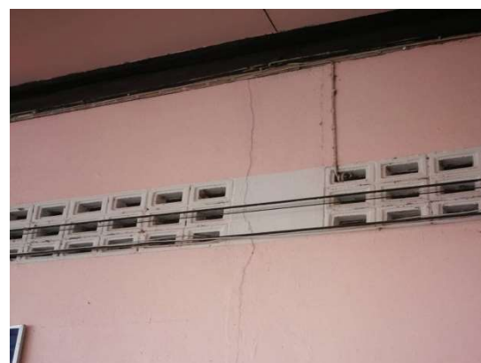
F-02: Vertical crack ( w=0.15 mm), condition rating = “Fair”
