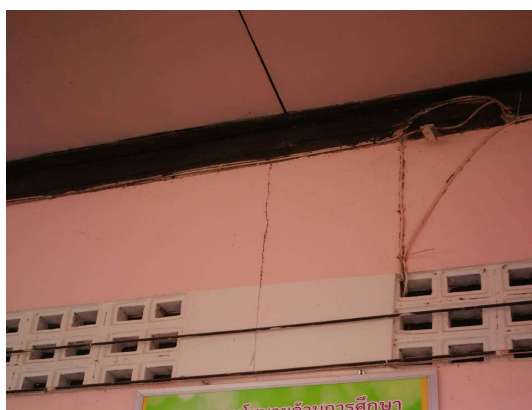
F-01: Vertical crack ( w=0.2 mm), condition rating = “Fair”
