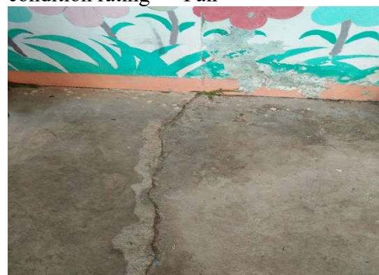
F-04: floor crack ( w > 2 mm), condition rating = “Poor”
